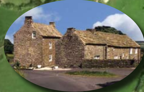
The defensive triangular formation of buildings at Woolley had high status in medieval Allendale
