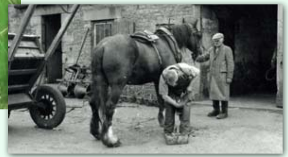
Thornley Gate Cottage had an adjoining forge (right, pictured in the 1960s) that was subsequently replaced by a filling station. Both are now demolished and have been replaced by a house.
